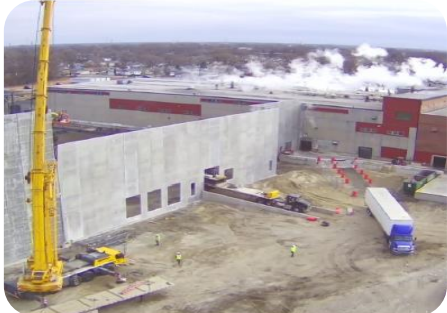
Construction Commenced December 2022
