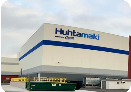
Construction Completed October 2023
